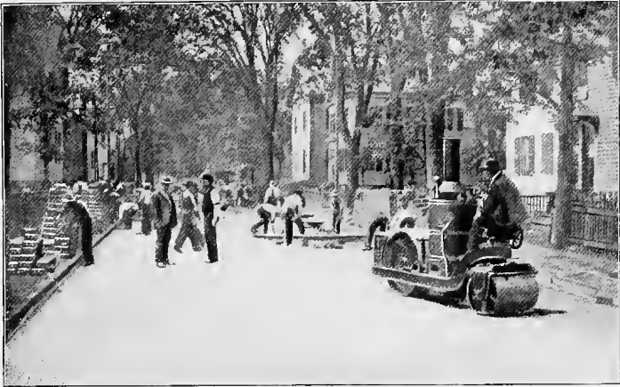
Rolling with two and one-half ton roller.
